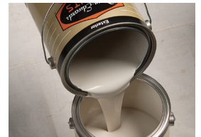
Intermix each new can of paint with some of the previous can for color uniformity.
