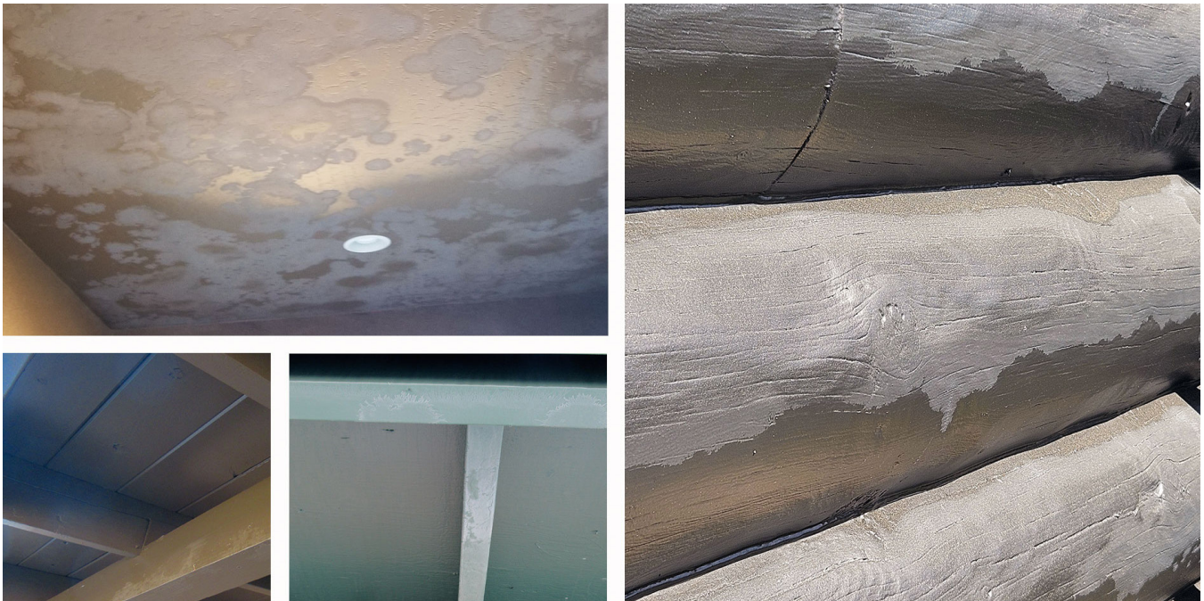
Figures 3 Examples of Surfactant Blooming on exterior surfaces.
