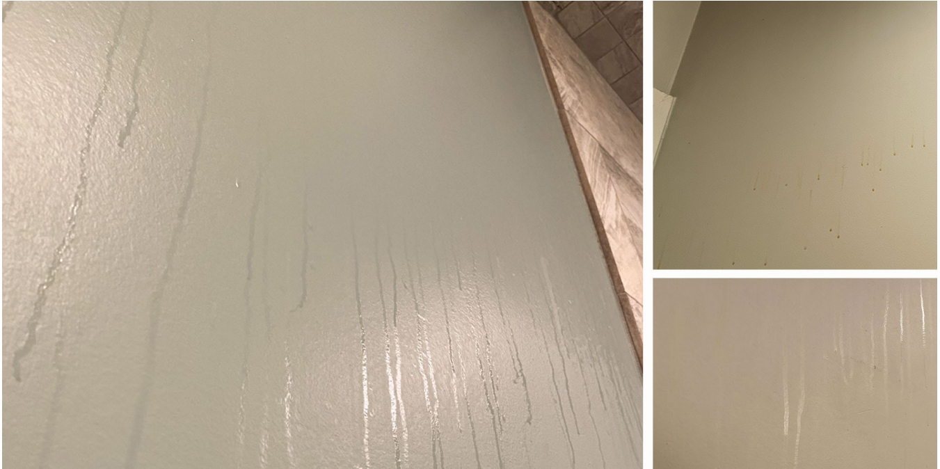
Figures 2 Examples of Surfactant Leaching on interior surfaces.
