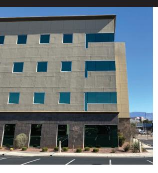
Finding the right primers was key as well. Vay's Dunn-Edwards rep suggested their FLEX-PRIME Select as a protective sealer with great bonding properties for the upper floors. The first floor of the building was built with concrete block veneer, a different type of substrate than the other three floors. It would require its own bonding patch coating, the Dunn-Edwards-sourced RAINGUARD Blok-Lok, used in many anti-graffiti applications.
