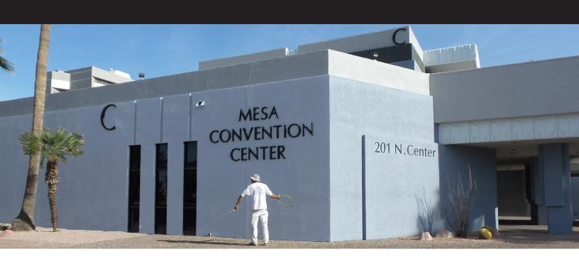
One recent project where that level of attention was key was the exterior repaint of the Mesa Convention Center and Amphitheatre. A variety of substrates across the properties called for a range of products including EFF-STOP Premium for priming masonry and Smooth BLOCFIL Select for priming block walls and planters—and ultra-premium paints: EVERSHIELD for walls and stucco, and ARISTOSHIELD for metal railings, doors and fences.
