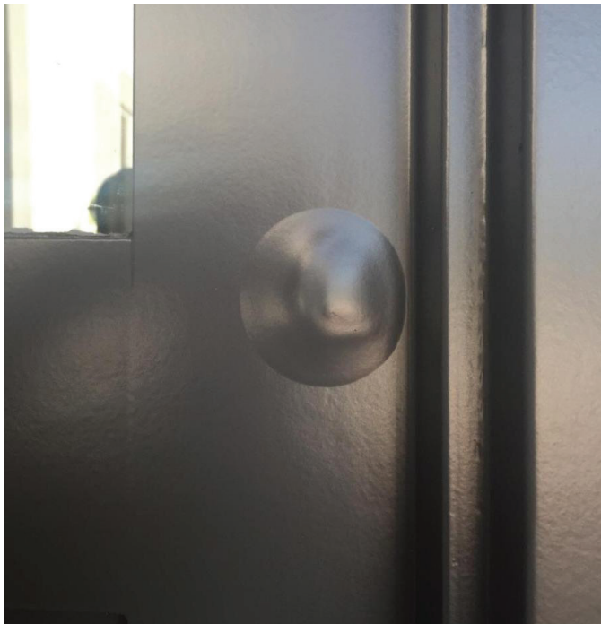
Figure 3: Blistering of dark colored paint.
